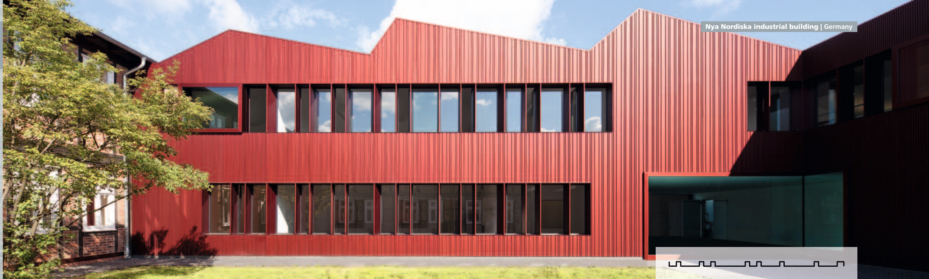
Irregular special profile SQ-20/20-R, AlMg1, Sandalor® anodised
