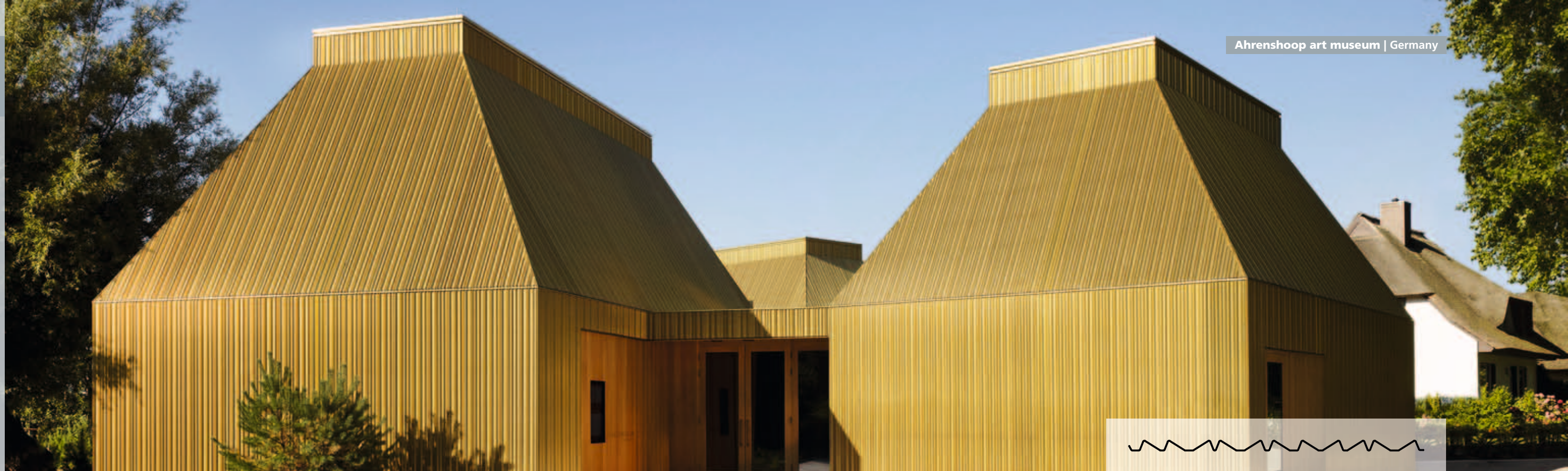
Irregular zigzag profile SZ-25/50-R, reflective, brass
