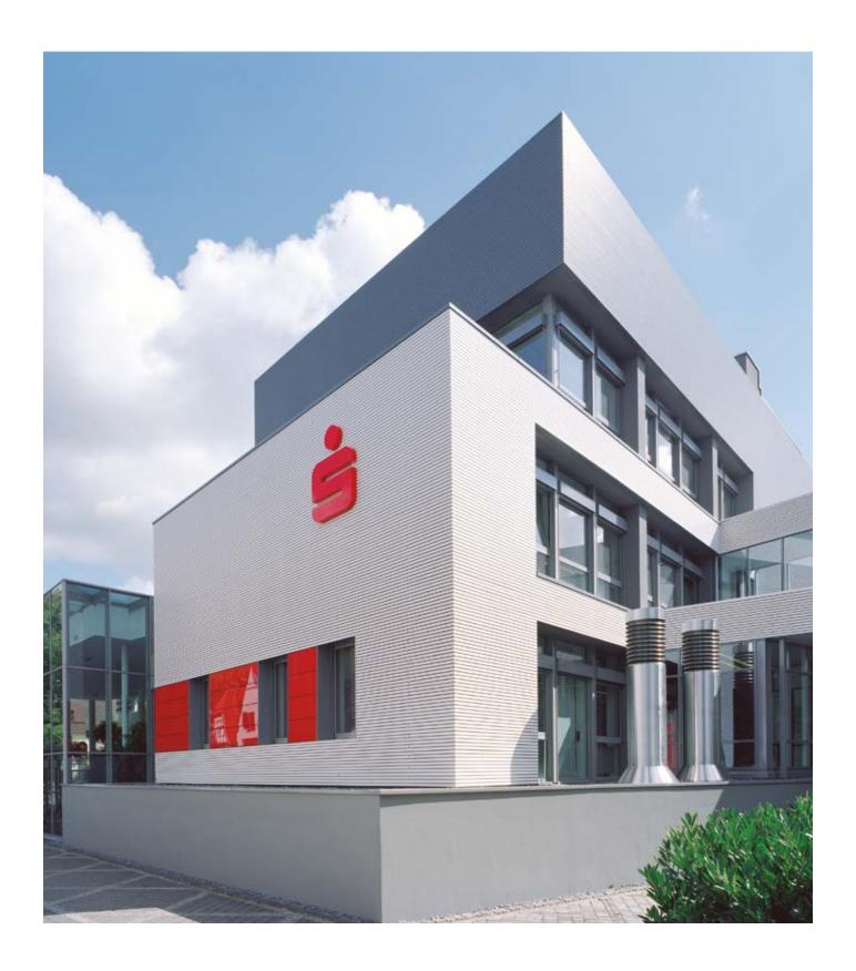
The Sparkasse in Rheda-Wiedenbrück is a good example of the high plasticity of the building elements, which is enabled by the Fshape aluminum façade system. This façade convinces with its extremely clean building edges. This is particularly apparent in the case of the building openings that spring inward. At the same time, this
