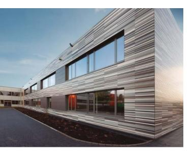
The rear-ventilated facade of Fshape is available in a variety of color design options. With this aluminum façade system, façades can be realized in simple gray tones as well as stronger colored accents. This lamella facade always emphasizes the cubature of the building. Both the protrusion as well as the recesses convince through the great plasticity and purity of the form.
